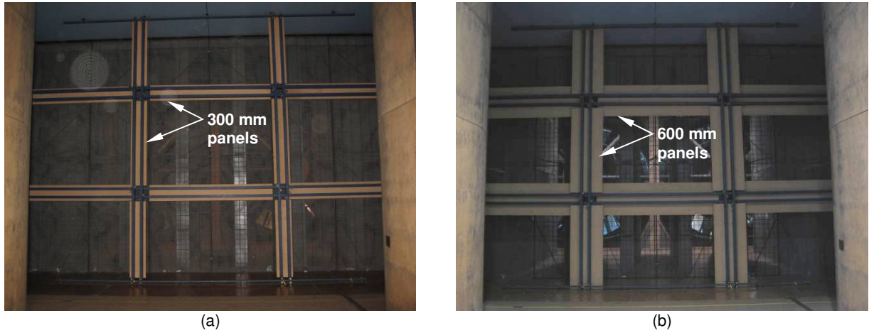
Figure 54: Grid installed with turbulence panels in the 12m x 5m tunnel section, just downstream of the fans: (a) 300 mm panels; (b) 600 mm panels.
