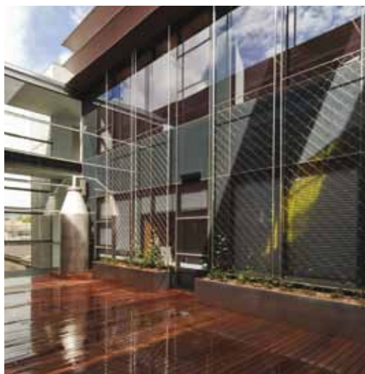
Building 9, School of Media and Communication.
